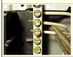
I stripped the insulation from the end of the wire and inserted the bare end into a connection terminal.
