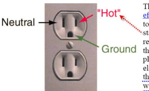
The high voltage (about 120 volts effective, 60 Hz AC) is supplied to the smaller prong of the standard polarized U.S. receptacle. It is commonly called the "hot wire". If an appliance is plugged into the receptacle, then electric current will flow through the appliance and then back to the wider prong, the neutral.
