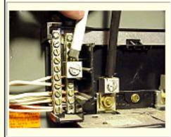
The neutral line feeding the panel is supposed to be marked white (this one was covered with white electrical tape, which is OK).
