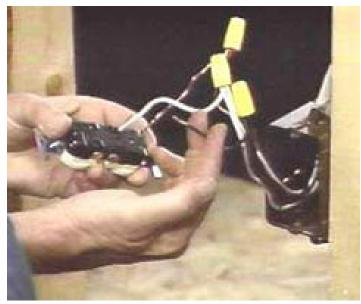
Connecting wires at a duplex receptacle. Strip all wires 3/4" and then hold all of the wires of like color together with another 6" wire of the same color. Twist the ends of the wires being connected with the pigtail wire tightly together. Then screw on a wire nut of the appropriate size. You can check the security of your connection by holding the wire nut and giving a good tug to each wire.
