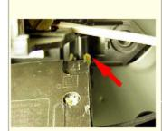
The installation sequence. First the hold-on clip is pushed onto the plastic bar. (I angled the breaker so a photo could be taken. In practice the breaker is parallel to its neighbor.)
