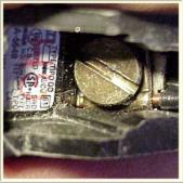
The hot wire was stripped and secured under the screw.
